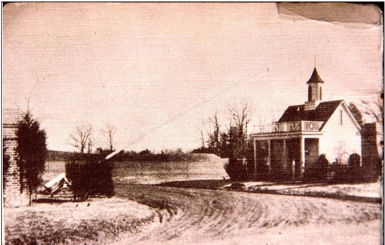
Figure 5-8. Gate walls and realty office, ca. 1928.
